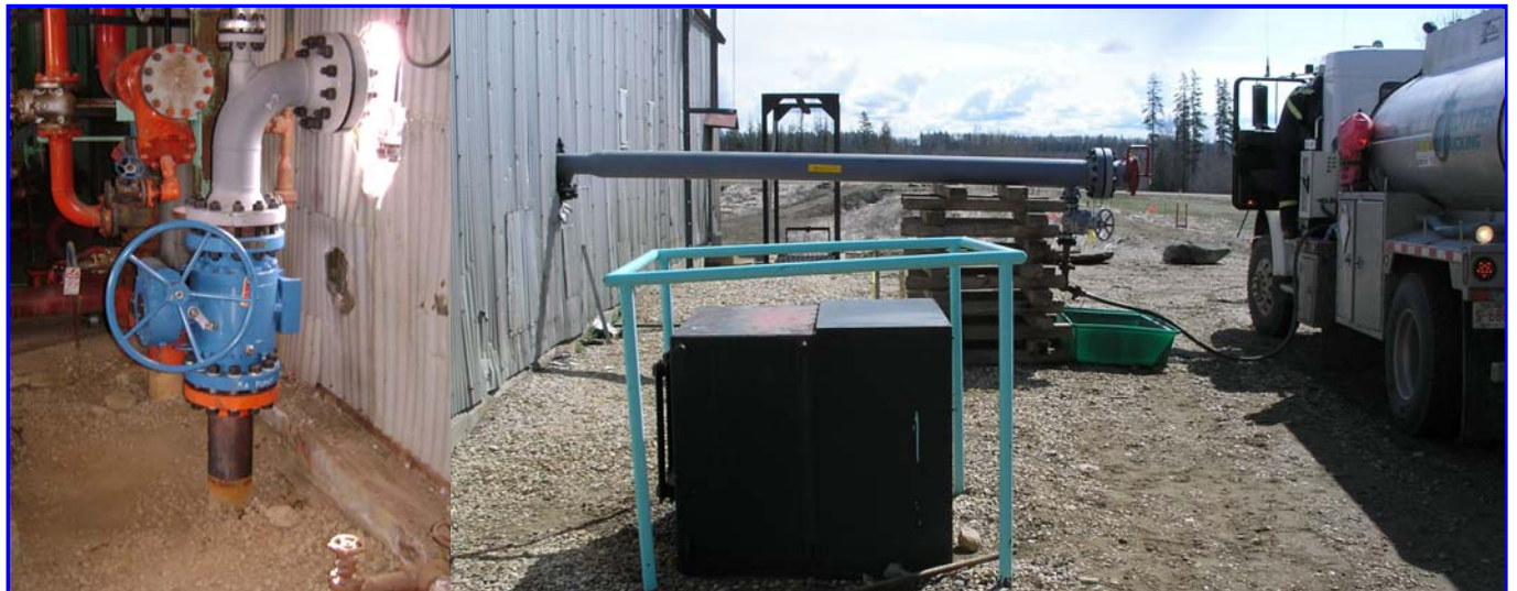
• Figure 5. Launch setup using pumper truck.
