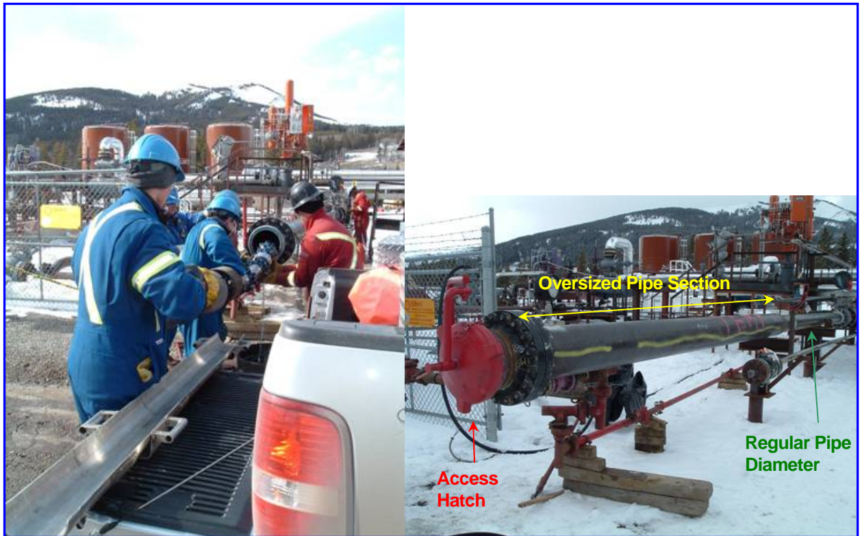
• Figure 3a. Tool insertion into Launch Barrel – 3b. Closed barrel after tool insertion.
